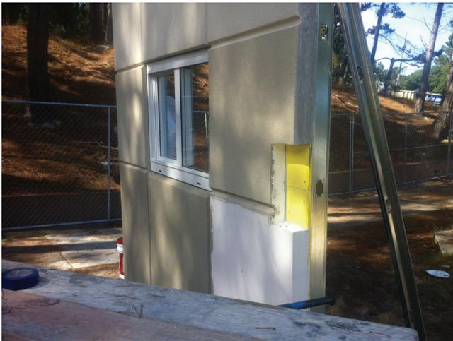
**Figure 7** PDQA process deliverables like window mock-ups can be effective quality assurance tools when used correctly.
