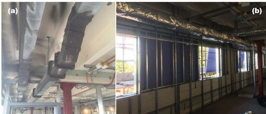
Figure 9 Ductwork joint seals (a) alone that did not meet DALT criteria and (b) insulation provided.
